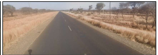
D869 Road Condition – Paved (Good)
