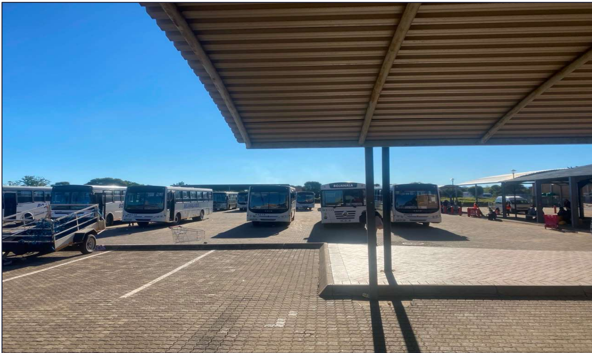
Figure 2-10: Bus facility in Northam Plaza Rank
