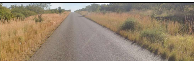
D1335 Road Condition – Paved (Good)
